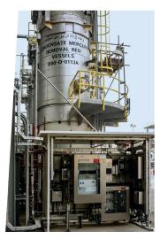
The Mercury Monitoring System MMS-NG is an ideal tool to determine the efficiency of each MRU in real time, and necessary to successfully monitor and control mercury concentrations during natural gas production and processing.
