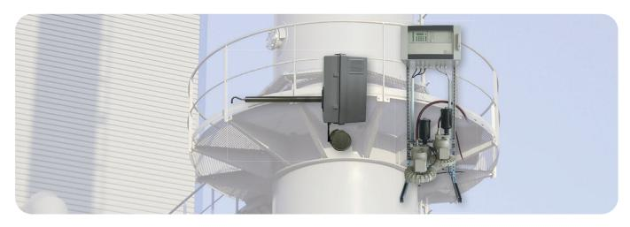
Continuous, tribo-electric extractive measurement of dust contents in wet and sticky exhaust gases
